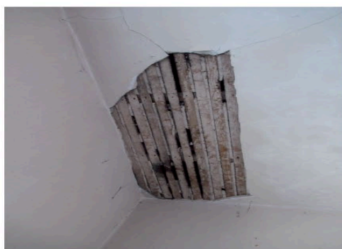
Figure 2.36 Lath and plaster ceiling exposed by loss of ceiling (Room 12.3)
