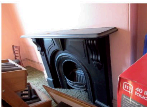
Figure 2.17 Typical intact timber surround fireplace with metal grate, located on the first floor (Room 2).
