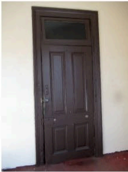
Figure 2.19 Victorian door (D34 in Room 4) with intact hardware and fanlight.
