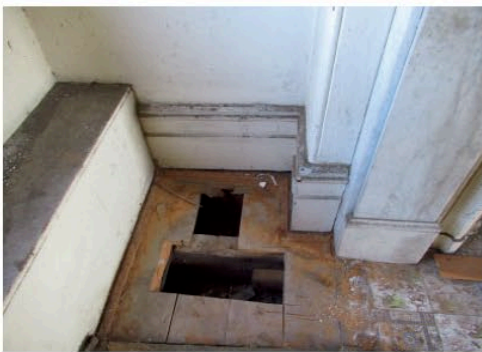
Figure 2.21 Tongue and groove timber floorboards on the first floor in Room 5.2.
