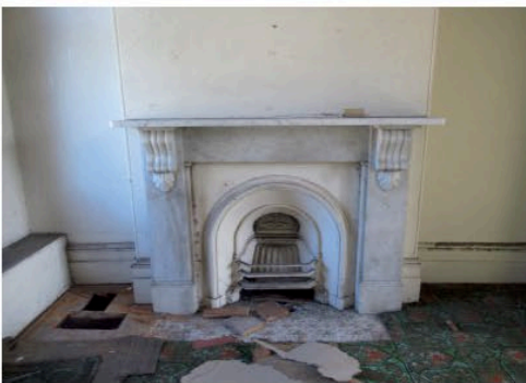
Figure 2.23 Typical intact original marble surround fireplace in Room 5.2 with metal grate and tiled hearth.
