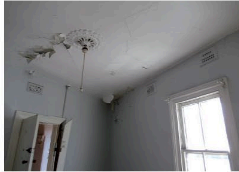
Figure 2.30 Peeling ceiling and wall in Room 11.1 with decorative ceiling rose.
