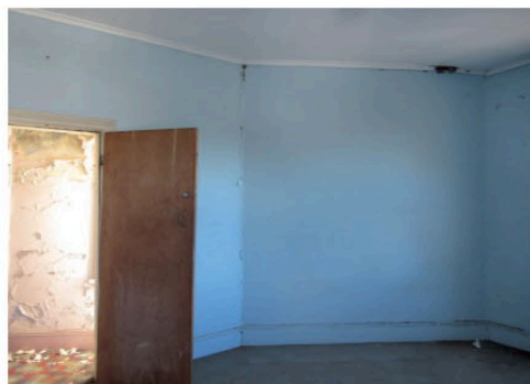
Figure 2.32 Termite 'mudding' to the cornice areas of Room 12.1, of the second floor.
