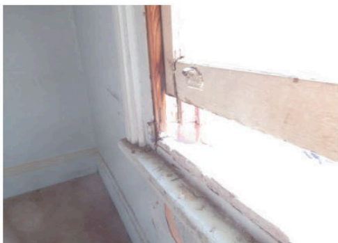
Figure 2.31 Damage to window sill (W42) in Room 8.
