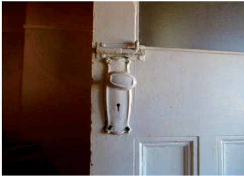
Figure 2.25 Inter-war high waist door with intact hardware in Managers Office
